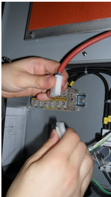
3 rd step: disconnect the heating plug connectors.
