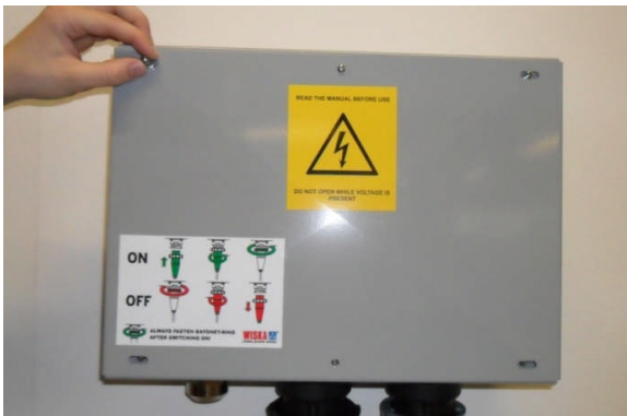
1 st step: undo the cap nuts.
